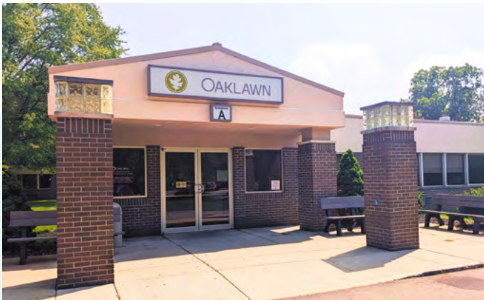
Elkhart campus (entrance)
